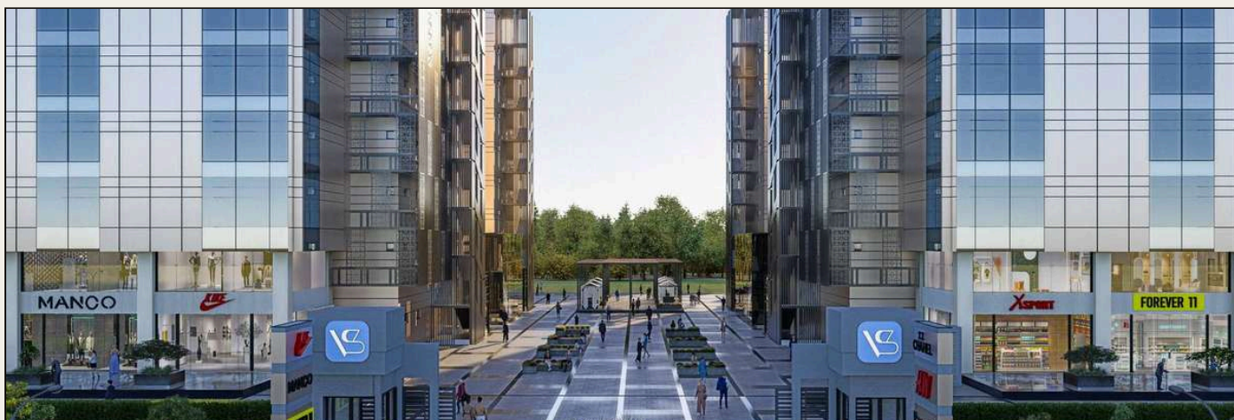
VISION BUSINESS PARK — THE ARENA OCCUPIES THE CENTRAL PLAZA
